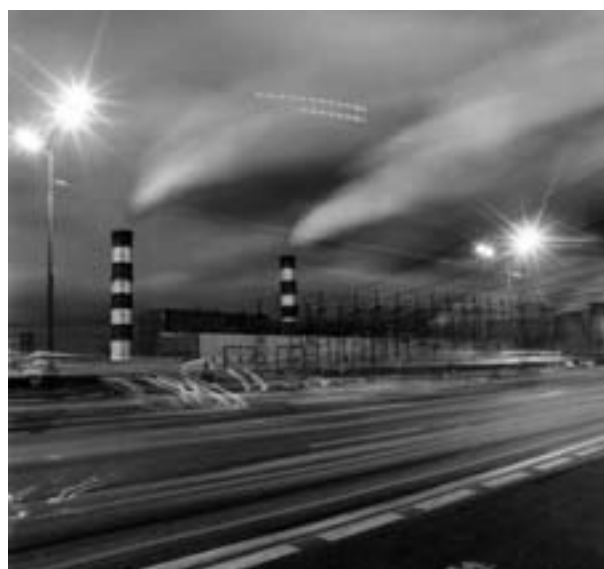
Traffic streams past the electrical power station beside Moscow's ring road. © PANOS/ Martin Roemers
